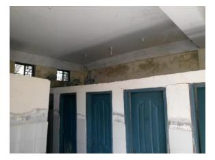
Heavy useless concrete mass at sun shade have been proposed and executed. It acts as water tank with draw down pipe at the bottom. There is no maintenance mechanism and all have been blocked resulting in the water storage and seepage into the walls of the hall.
